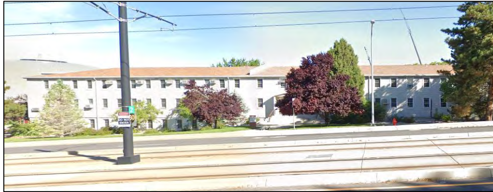
VIEW TO THE NORTH
