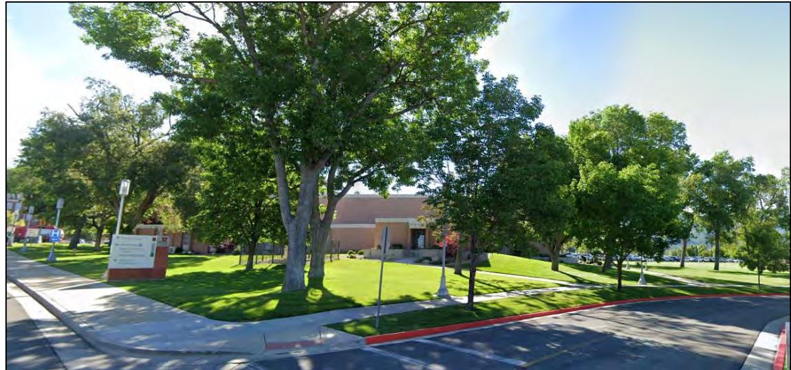
VIEW FROM THE WEST
