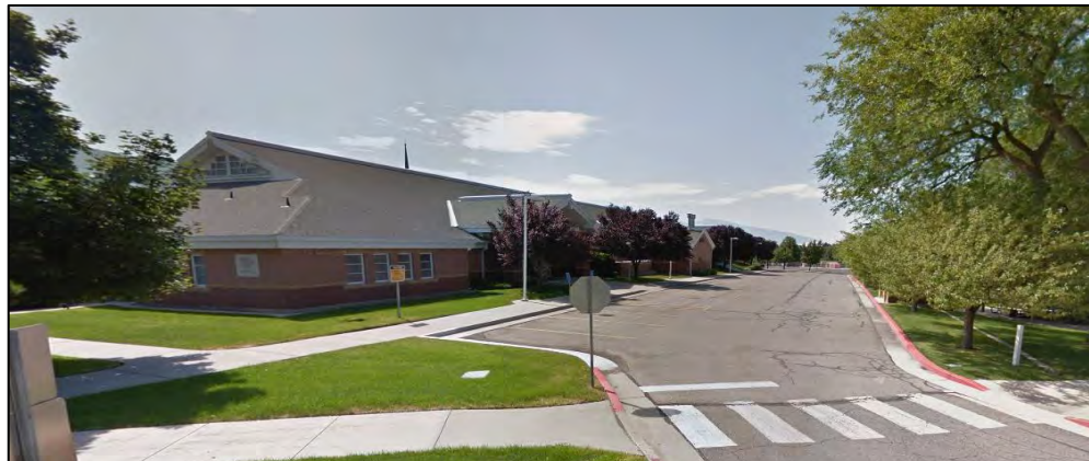
VIEW TO THE SOUTH
